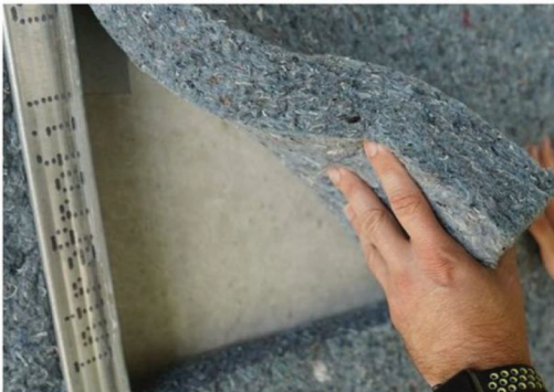
Recycled textile insulation in use
